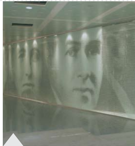
The Illinois Institute of Technology in Chicago features silkscreened glass from Goldray Industries, Calgary, Alberta. In addition to silkscreen/screen-printed products, the decorative glass supplier offers traction control frit for glass flooring, opaque coated glass cladding, satin etch translucent glass, decorative laminated glass, technographic interlayer, tempered and fabricated glass and doors, and glass marker boards.
