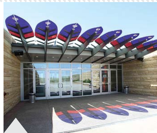
The Eagle Feather Fan at the front entrance of the Blackfoot Crossing Historical Park in southern Alberta, Canada, features decorative laminated glass from Lami Glass Products, Vancouver, British Columbia, a division of Hartung Glass Industries. Lami Glass offers Impact decorative laminated glass that combines the structural safety and security of laminated glass with the brilliant color of film. In addition to exceptional strength and acoustical characteristics, Impact provides users the ability to create unique glass combinations by laminating different layers of films, colors, textures and patterns into a single lite.
